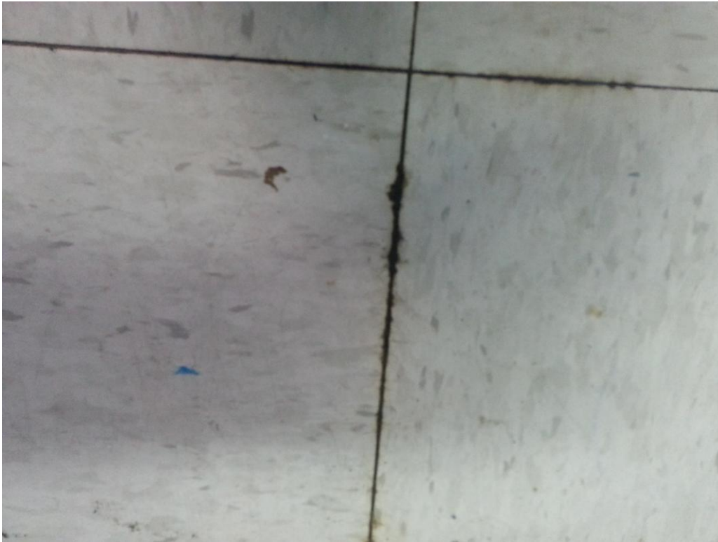
Black material on floor tiles is dissolved glue from underneath, elevated moisture bedside window
