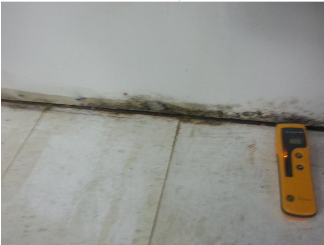
Standing water on floor of HVAC room, wall with mold is on other side of the brick wall, visible mold on base of wall in classroom, moisture about 17%
