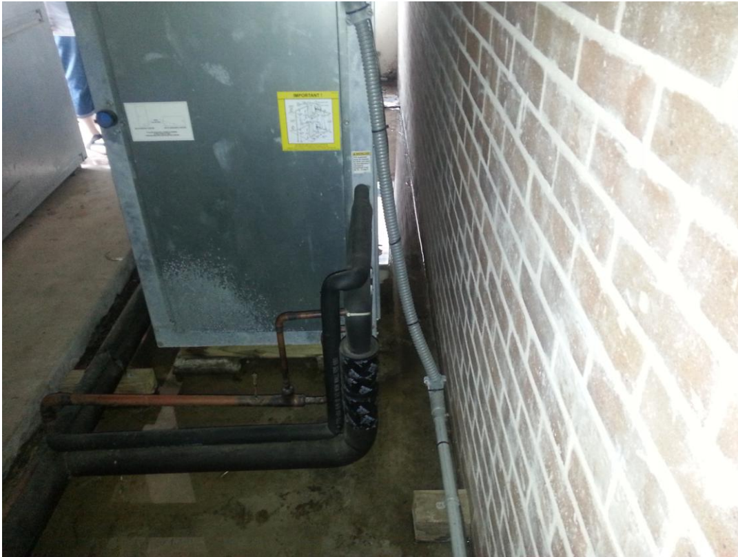
Standing water on floor of HVAC room, wall with mold is on other side of the brick wall, visible mold on base of wall in classroom, moisture about 17%
