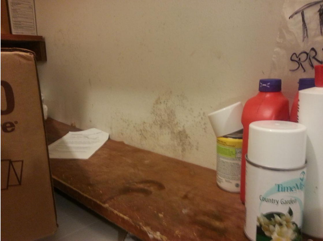
Moisture level 18% in exterior wall, mold on wall in janitor's closet
