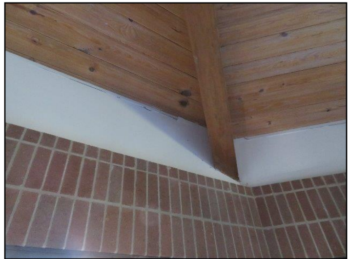
29. Water damage
