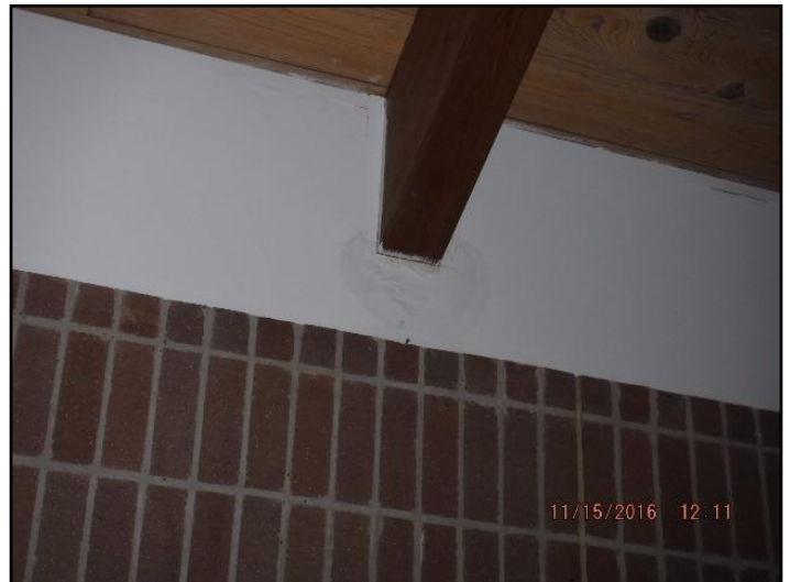
33. Water damage
